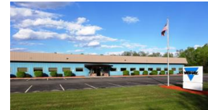
Dover, NH Vishay HiRel Military / Avionics / Industrial
